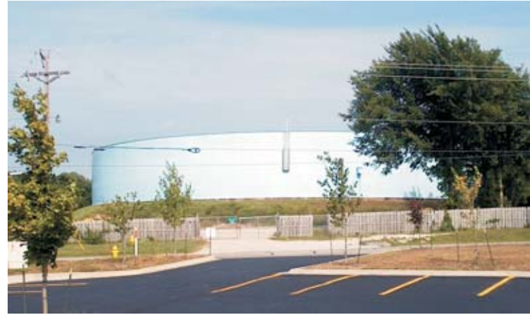
Chipman Road (High Service) Ground Storage Tank
